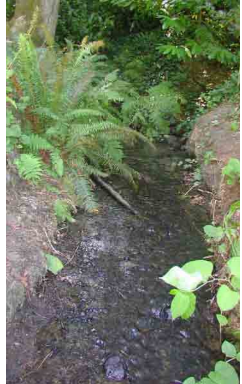
FIGURE 1.10.-- Photos of Scheuerman Creek (stream system #21). The left photo was taken at the creek mouth where it exits a culvert and then drops sharply to Puget Sound. The right photo of Scheuerman Creek was taken approximately 30 m upstream of the culvert and shows the overall shallow depth of this stream.
